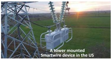
Figure 5 - Smartwire Device Installed on Overhead Line
