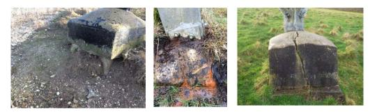
Figure 11. L-R – a) Exposed Foundation, b) Corrosion of Embedded Steelwork, and; c) Significant Cracking through Muff Concrete
