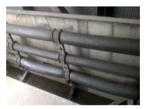
Figure 7: Bulging cable showing damage to cable sheath
