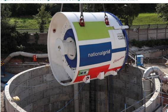
Figure 5.7 Tunnel boring machine being lowered into a vertical shaft
