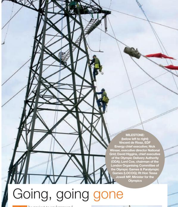
he project to underground National Grid's electricity supplies running across the 2012 Olympic Games site is due to complete in December with the dismantling of all 29 pylons on the now redundant 275kV overhead line between Hackney and West Ham substations.
